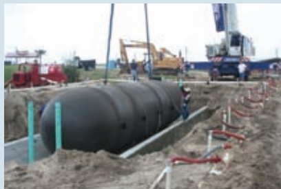
Tank Installation at Sunset Cove in Galveston, TX
